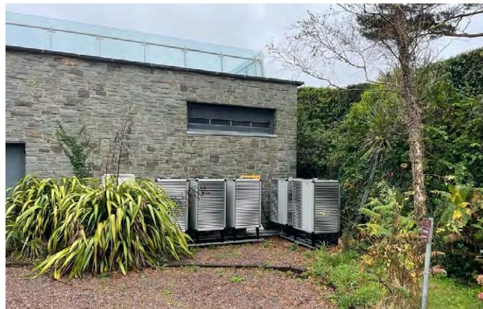
The modernisation of the heating and domestic hot water system at Parknasilla Resort & Spa has resulted in significant energy savings. By replacing the LPG gas boilers with a Master Therm heat pump system with intelligent control, the leisure centre has become significantly more efficient and sustainable in the long term.
